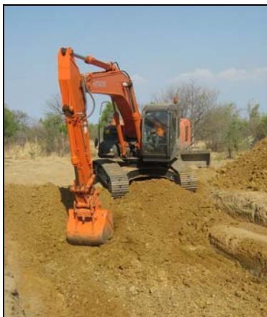
Langey Costean Excavation
