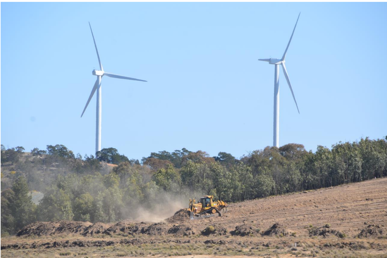
Figure 3: ROM pad top soil removal.
