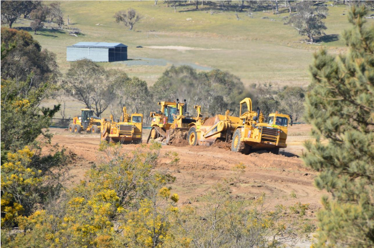
Figure 2: Pad levelling over the plant site.
